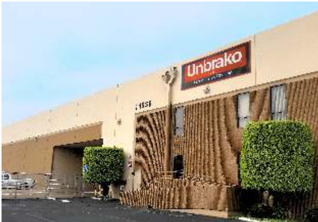
West Coast Distribution Center
